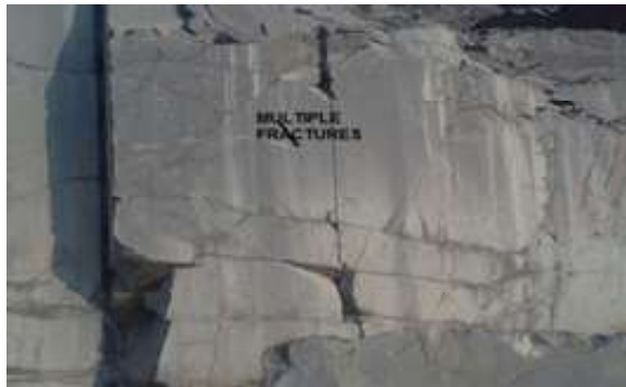
Fig 6. Multiple, fractures in granite quarry
