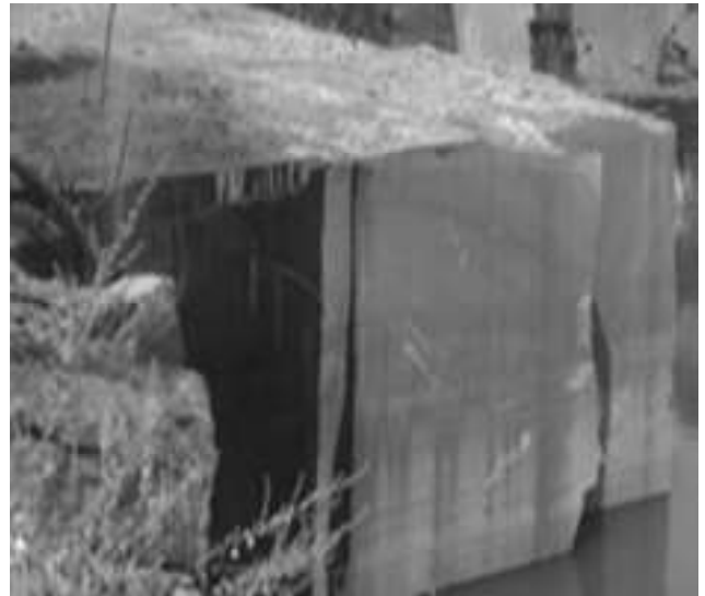
Fig. 4. Favorable vertical joint in dolerite rock deposit, Warangal, Telangana state
