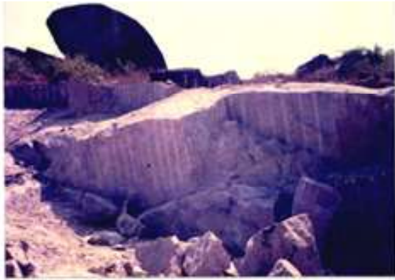
Fig 5: Unfavourable joints resulted in a huge waste in granite quarry during blasting in Karnataka
